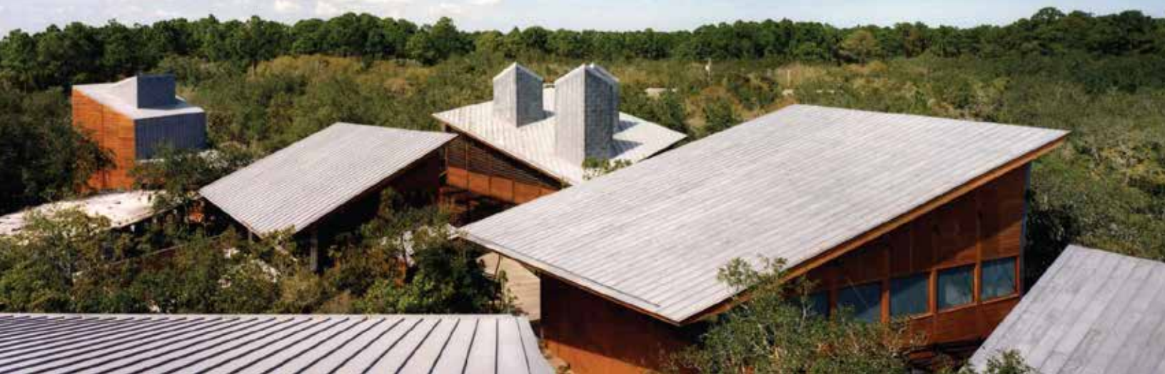
The Leeper Studio Complex at ACA Photo credit: From the archives of Atlantic Center for the Arts
